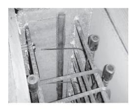
The joint sealant is applied to the middle of the construction joint. It is advisable to allow at least 8 cm of concrete on both sides of the expanding sealant to prevent cracks in the concrete.
